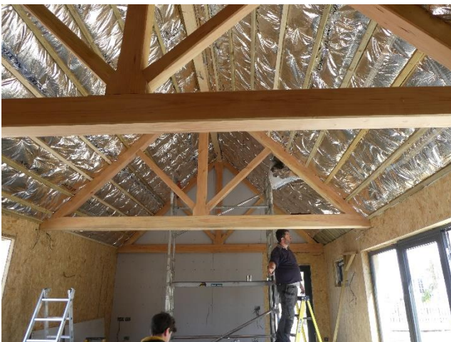
15 th April 2020: all the fire retardant and insulation in the roof is in place followed by plasterboard before painting.
