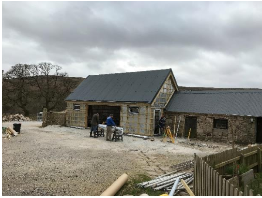
2 nd April 2020: doors and windows with dark grey metal frames are inserted. Takes a while!
