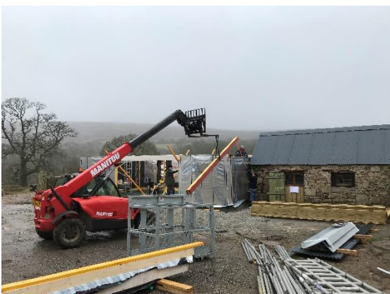
17 th -18 th March 2020: beams go across to add security to the frame.
