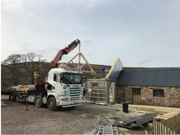
20 th March 2020 – the trusses made with secretly inserted metal joints are carefully lowered into position.
