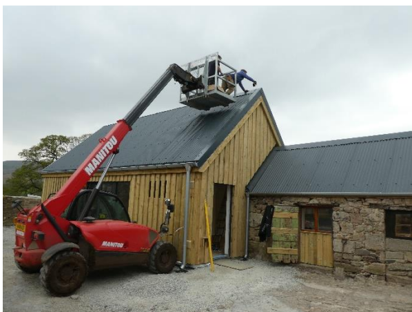
27 th April 2020: Tristan and Ed use a spray on adhesive to secure the 'wavey' foam ridging material that holds on the final ridge pieces which are drilled securely in place.
