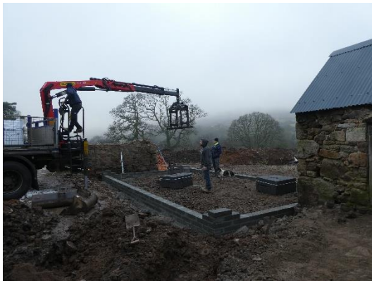
22 nd January – the blocks arrived and the foundation walls are built by Matt and his brother.
