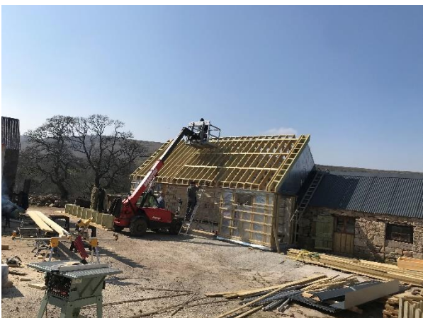
24 th March 2020: Will deftly manipulates the Manitou speeding up the roof work and enabling considerably faster work than would be possible with scaffolding.
