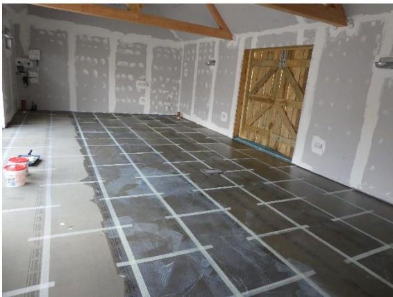
19 th May 2020: special underfloor heating mats are laid and sealed with tape by Ed over the hard chip board.
