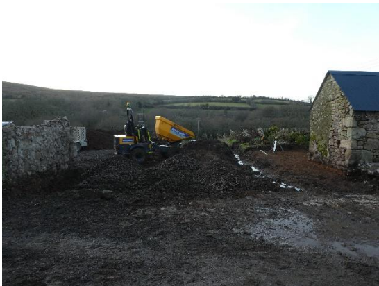
15 th January: main drains dug and foundation gravel laid.
