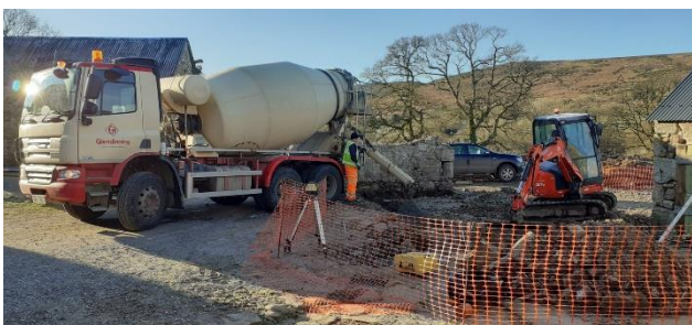
21 st January 2020: Glendenning's delivery of cement for level one of the many foundation levels.
