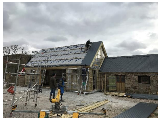
30 th March 2020: first layer of breathable membrane Followed by the anthracite covered metal sheeting.
