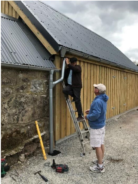
13 th May 2020: Malcolm and Dave visit for a day to install the guttering on the Corndon side to the office and the drain pipe for the two buildings.
