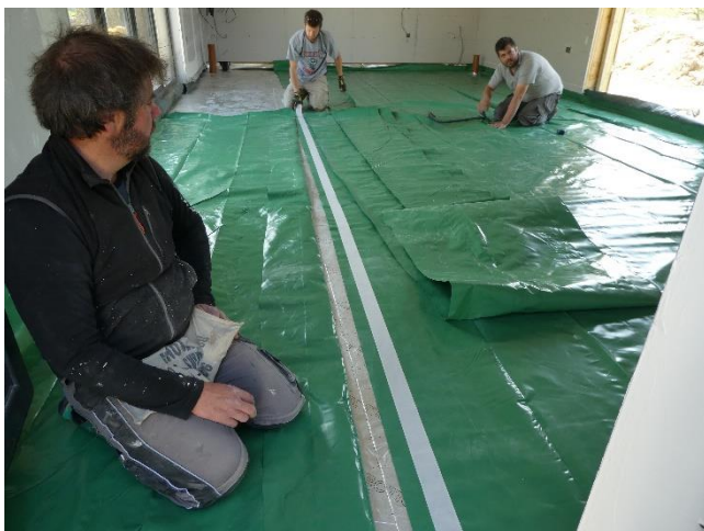
22 nd April 2020: all joins are carefully sealed with tape for both the radon barrier and the Celotex.
