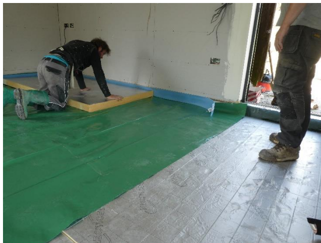
22 nd April 2020: A second radon barrier is placed between the two layers of Celotex, with a damp seal lining around the edge.
