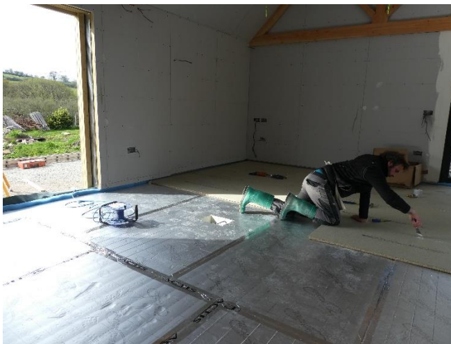
22 nd April 2020: more sealing and more securing of specialised hard chip floor boarding'
