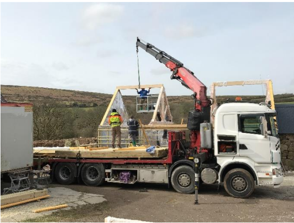
20 th March 2020: machines on both sides to ensure people are in place to secure the roof beams.
