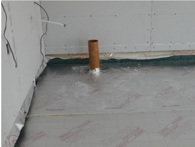
22 nd April 2020: all seals are carefully taped and snugly fitted to ensure no leakage of air, moisture or radon.
