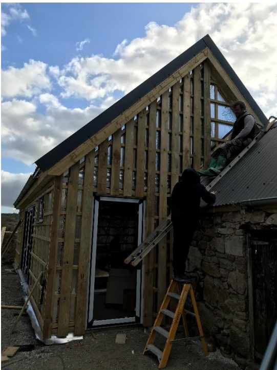
6 th April 2020: the outside boarding in 'standard' farm boarding (hit and miss boarding) has begun.
