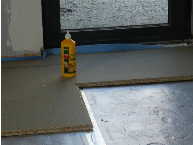
22 nd April 2020: 22ml chipboard is placed and sealed over the Celotex.
