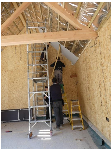
20 th April 2020: the first roof plasterboard is hoiked up and held in place as the screws are drilled. It's a four-person job, with very tired arms and necks at the end of the day.
