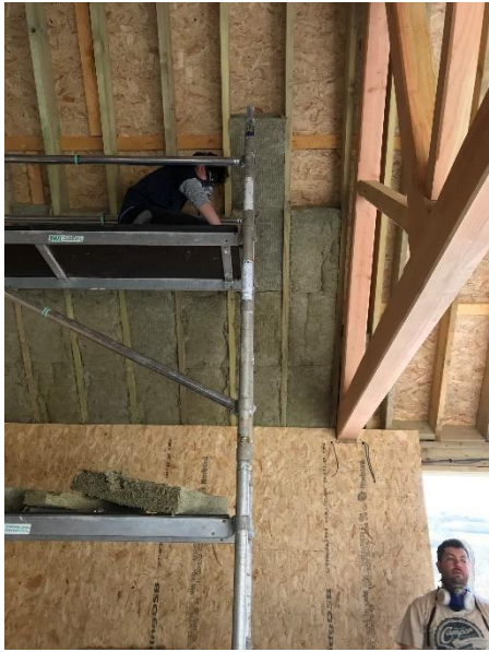
8 th April 2020: Rockwool under the hardboard is followed by layers of thermal insulation, fire retardant and yet more boarding. It will be very warm!
