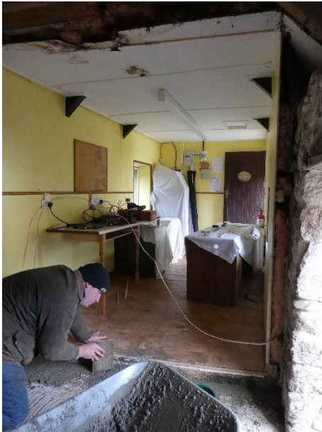
15 th November 2019: Will Dracup, our Farm Manager sets to work cementing the gaps where the rats have been active under the office for the last twenty years or more!
