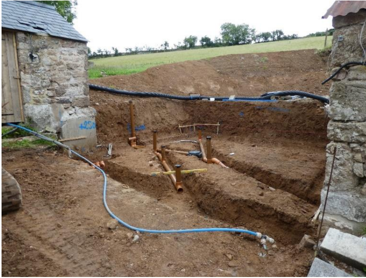
July 2020, carefully laid ducts and pipes to receive water from our own borehole for filtering as tap water and heating in the Barn and Boot room.
