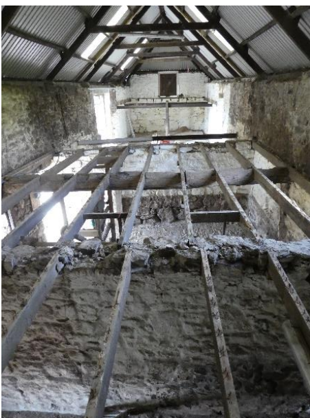
May 2020: volunteers had removed all the internal wood, preparing the space ready for future work, a new roof, new floors, insulation, new drains and heating.
