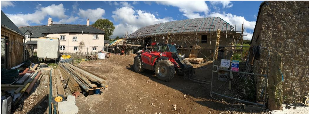
29th September 2020: View of the yard with the Tyvek waterproofing on the Barn roof awaiting new metal sheeting.
