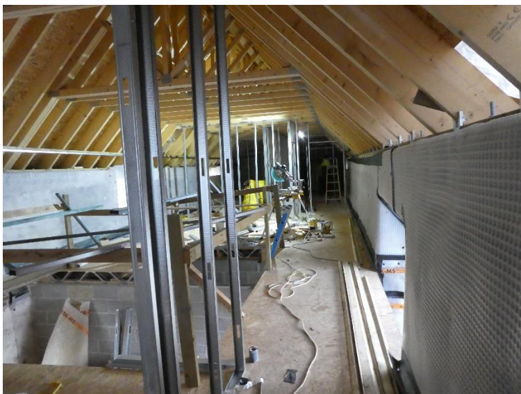
6th October 2020: PermaSEAL wall tanking to enable any condensation or damp seeping through the porous granite to trickle down to drains in the floor keeping the walls ventilated and dry. Celotex and rockwool were secured for insulation, covered by hardboard and a final layer of plasterboard before painting.
