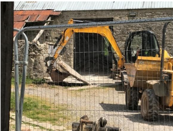
18 th May 2020: The first equipment to arrive was harris fencing to cordon off the area for security and insurance purposes. On day one of the diggers arriving, the cement was lifted to allow easy access and ensure internal and external 'levels' could be corrected.
