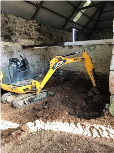
22nd May 2020: the priority was to determine what rocks lay below the floor in the Barn, which needed underpinning and damp proofing.
