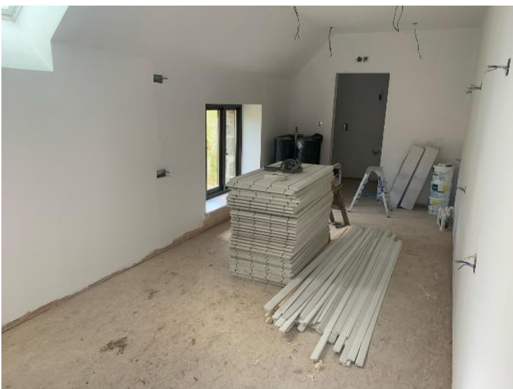
8 th January 2021: Room Five, the same room in which there is a bunk bed (picture above), fully boarded, plastered, first fixings of electricity and one coat of paint. Note the painting was undertaken by volunteers. THANK YOU!!!
