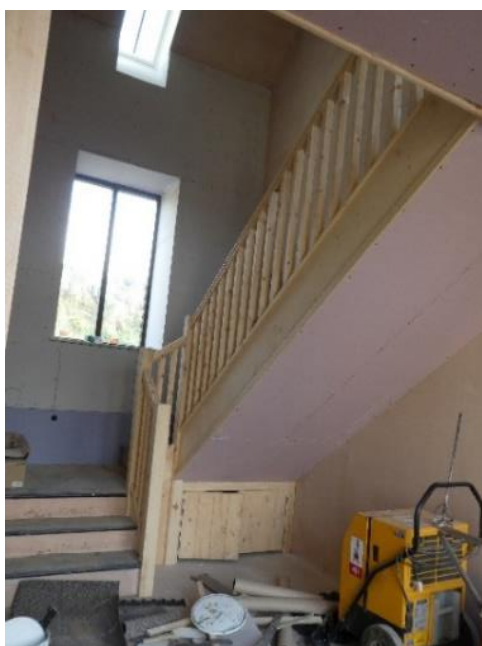
8 th January 2021: the stairs have been installed with close spindles to ensure good safety and wide steps to ease the flow of people.
