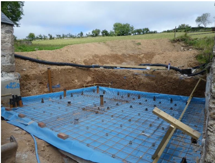
15 th July 2020, the damp lining had been laid.
