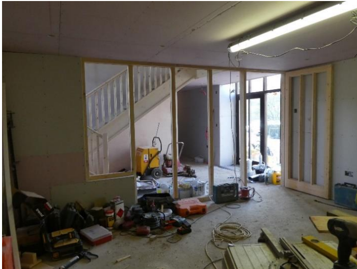
13 th January 2020: view out of the dining Room towards the main Barn entrance. Glass would be installed in the timber frames as the room has no other windows due to Grade II planning restrictions.
