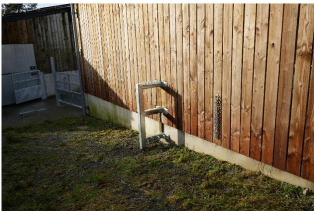
Holding mounts for the Farm Yard gates: December 2023. The gates are too heavy to be moved by the general public, but the ability to remove them enables a more diverse space.
