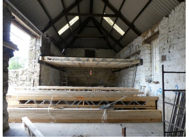
July 2020, the first floor is drilled into the sturdy ancient walls before the multiple layers of insulation were applied.
