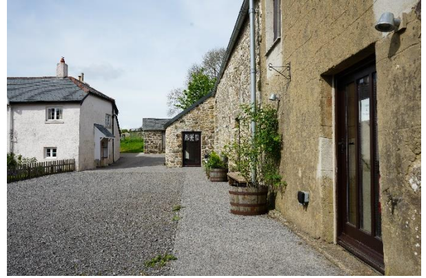
May 2024: A new cement path was laid with gravel to help the flow of rainwater and access through the yard. New glass doors replaced the old stable wooden ones to allow light into the building.
