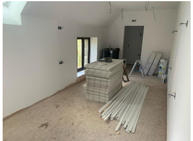
8 th January 2021: Room Four, fully boarded, plastered, first fixings of electricity and one coat of paint. Note the painting was undertaken by many volunteers. THANK YOU!!!
