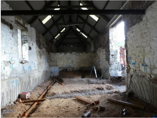
June 2020, all the old beams and wooden structures were removed, the floor levelled and drainage channels dug.
